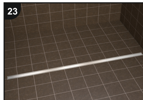
Griglia Double Face montata con la superficie in alluminio lucida in vista. In this view Double Face grid's polished aluminium side is mounted.
